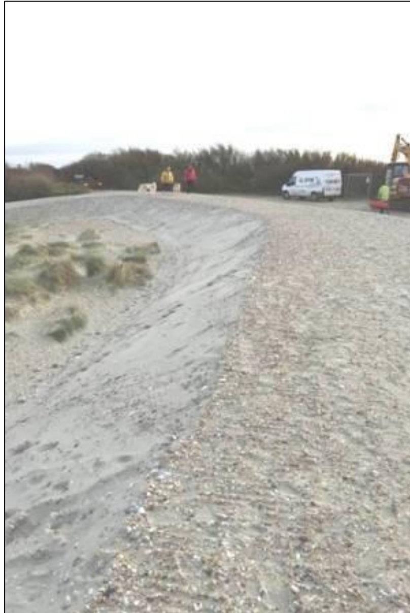
Figure 5.1 Sand and shingle ridge constructed along the back of the hinge, designed to reduce the impact of overwashing during severe storms (CHC, 2016).
